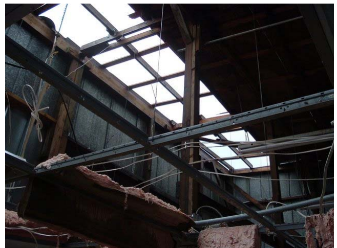
CEILING/ROOF OF CRATE AREA
